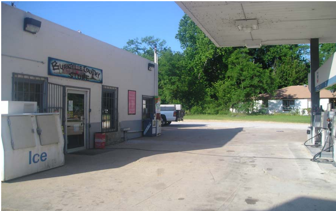
Photo 1: View facing west of Burnsville Country Store. Pump island on the right side of the picture. Tank pit also seen on the right side of the photo.
