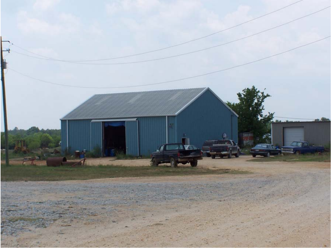
Photo 3: View of the building at Scott's Trailer Wash.
